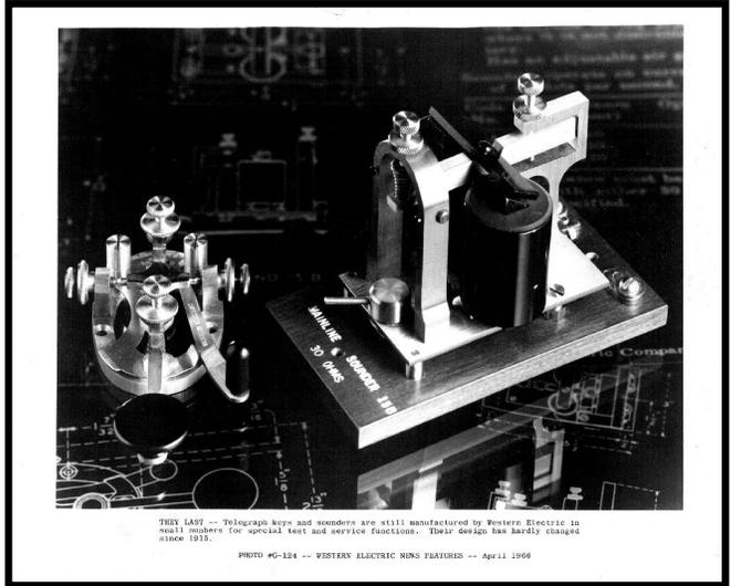
THEY LAST -- Telegraph keys and sounders are still manufactured by Western Electric in small numbers for special tests and service functions. Their design has hardly changed since 1915.
